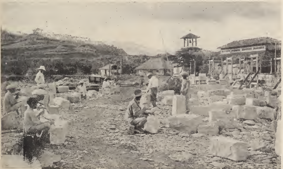
CUTTING THE STONE FOR THE NEW CHURCH.
